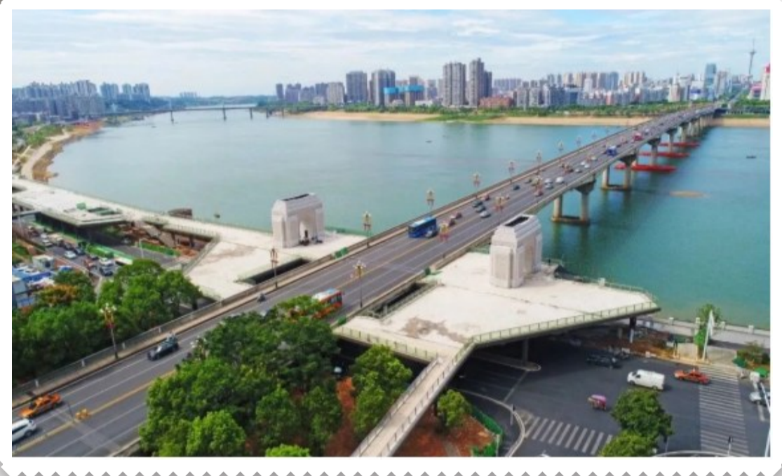
▶株洲大桥桥东今貌
