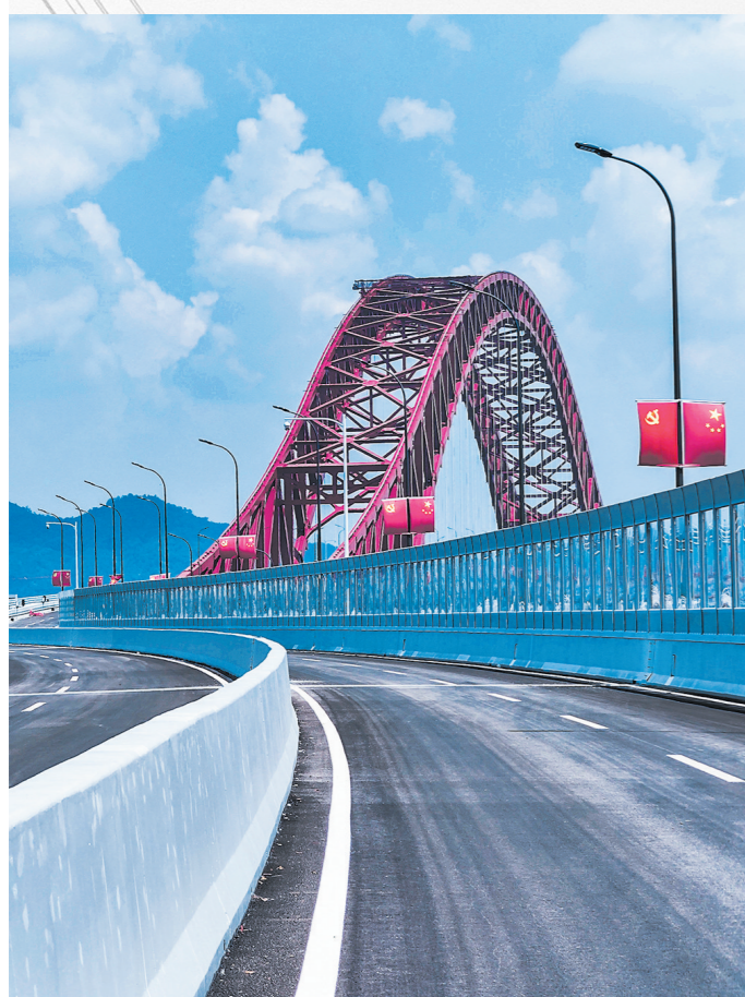
稍远处观看大桥,刚架开齐
